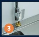
Push the tap body on and tighten both grub screws to finish.
